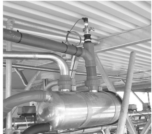
**Rotary Dairy** – mount as close as possible to the gland, in the installation photos below the tee moves the transducer out of direct air flow – this is good. There is often a spare outlet in the gland this is a good point to mount the transducer – beware of the transducer being accidentally knocked by operators or moving pipe work. If possible always mount the transducer upright to protect against moisture ingress.
